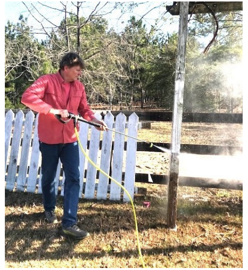
Rich Byer power washes the arbor.
