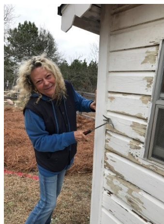
Leslie Platt scraping peeling paint off the playhouse.
